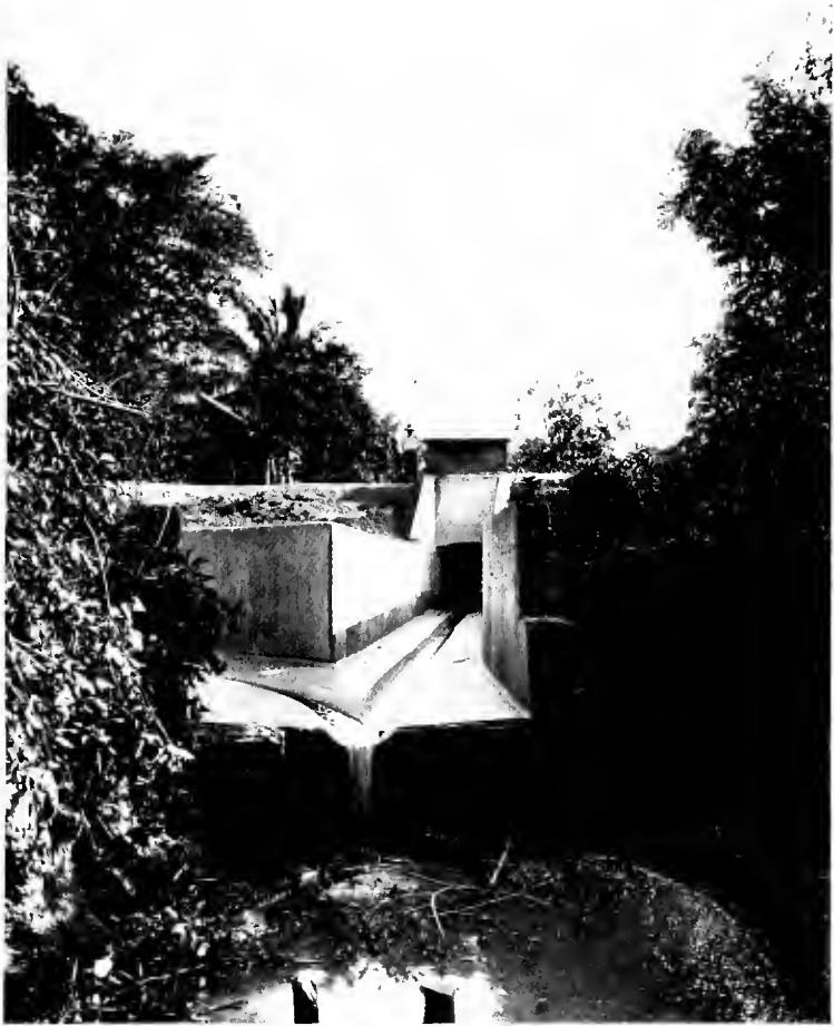
FIG. 28.—LARGE CONCRETE DRAINS, PORT OF SPAIN, TRINIDAD.
